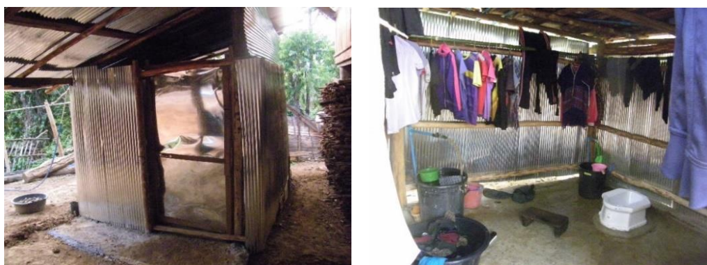
Latrine/shower units in Ban Yod Pai
